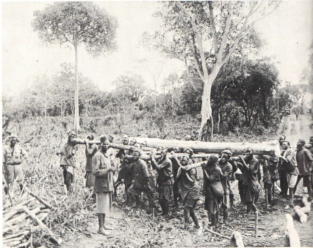
African Pioneers of the 2nd Road Corps manhandle tree trunks cut down in the bush for use in bridge-building. The Pioneers' unstinted enthusiasm made up for their lack of equipment.
